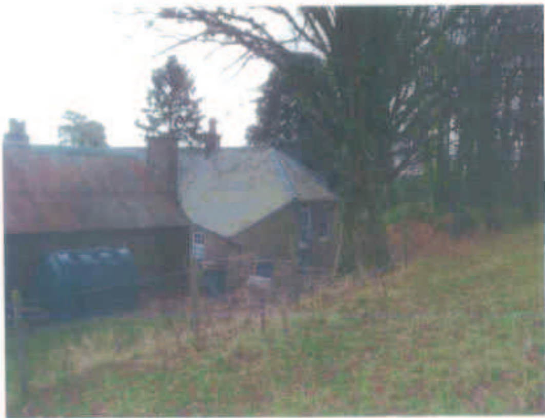
Fencing obstructing access into Tyle Gwyn Farm
