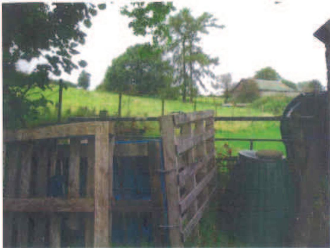
Obstruction preventing access onto Mr. and Mrs Tiley's ground where the right of way crosses and then enters into field through fenceline.
